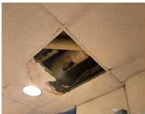
Above: Outside Cafeteria Submitted: September 27, 2021 Last District Update: October 13, 2021- Tile has been cut to remove mold, light is supported by rest of tile, if remaining tile is removed light will have to be disconnected
