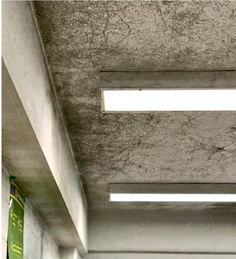
Photos 4 & 5 – Mold Growth on Ceiling and Wall of Occupied Elem. Classroom - according to teacher, condition present for months — Associated with HVAC System Problems
