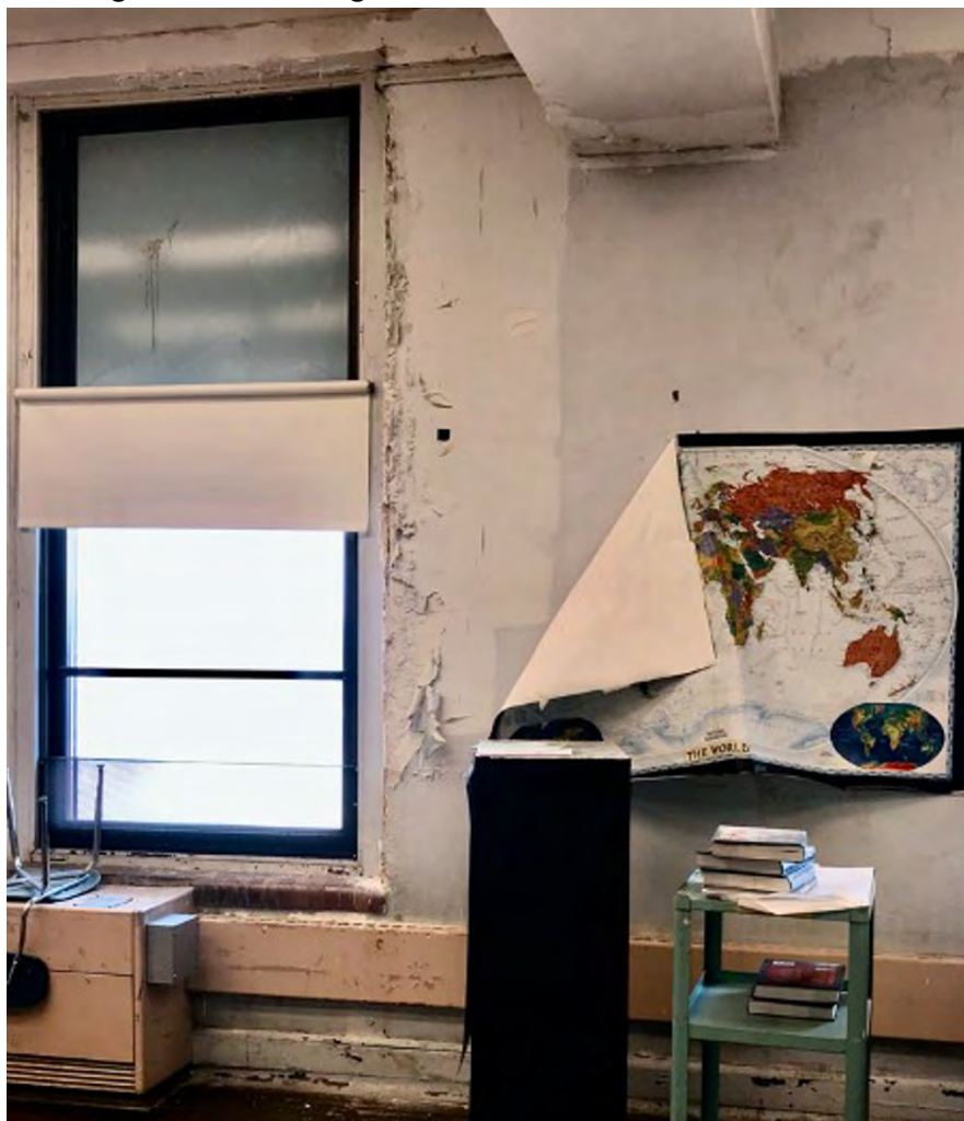
Photo 1– Elem. Classroom — Antiquated classroom unit ventilator, damaged/flaking lead paint, and obvious signs - and damage associated with - moisture and water intrusion.
